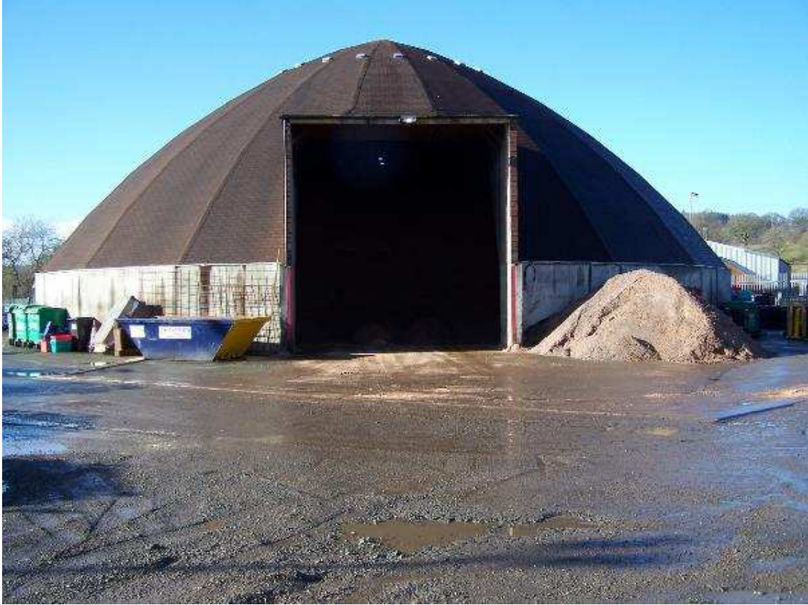
Dome Uk Salt Dome, PCC Welshpool Depot
